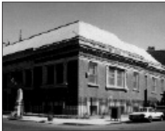
Large windows on facades at Macon Branch
