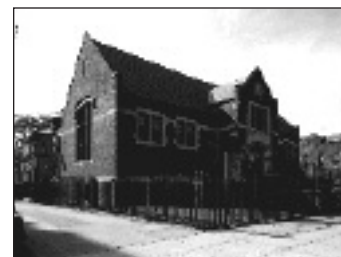
Steeply pitched slate roof at Washington Irving Branch
