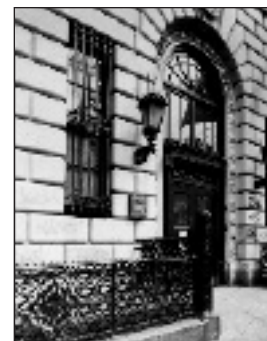
Lighting at entry of Hamilton Grange Branch (NYPL)
