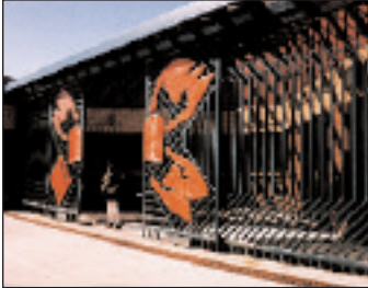
Decorative exterior gates at Cypress Hills Branch
