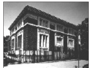
Perimeter fencing at Bedford Branch
