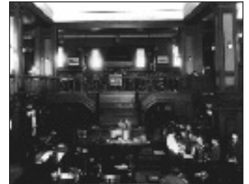
Interior of Arlington Branch with integrated perimeter and freestanding stacks (historic photo)
