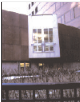
Cladding at Brooklyn Heights Business Library Addition
