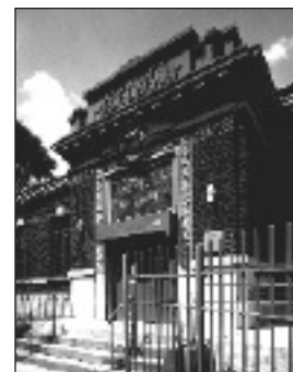
Entry at Saratoga Branch in need of restoration
