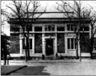
Bedford Branch (historic photo)
